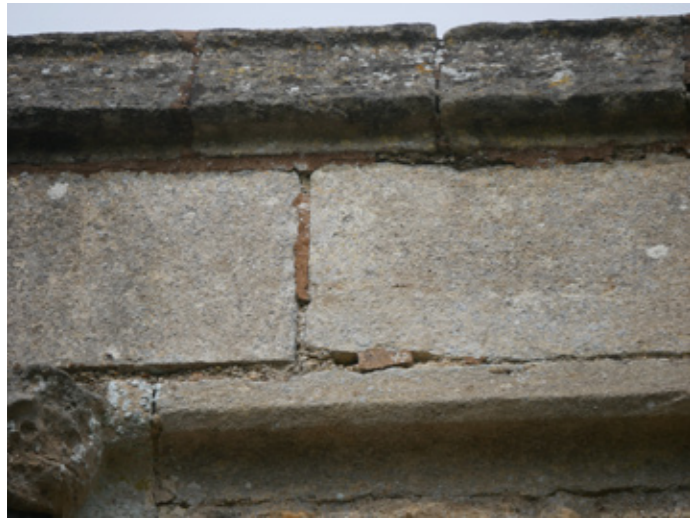
P17 South Aisle South elevation parapet
