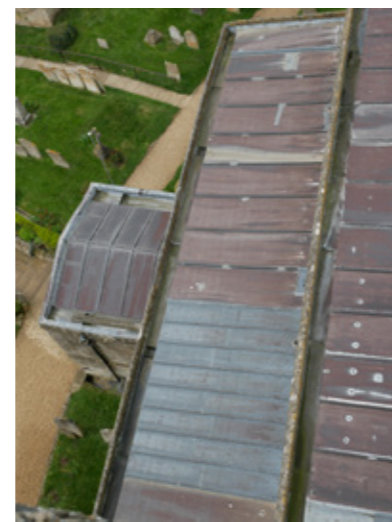
P06 South Aisle roof
