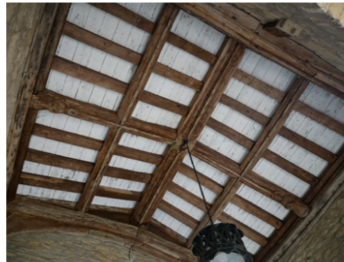
P35 Porch ceiling
