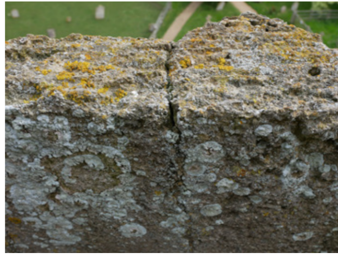
P02 Tower East parapet coping
