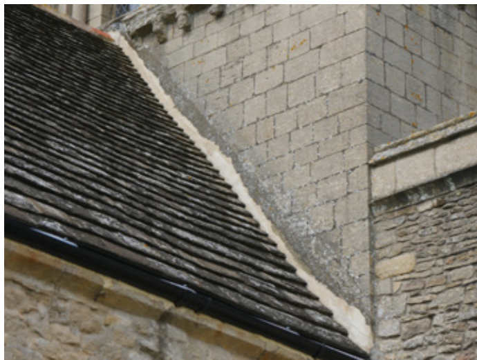
P05 South Transept East slope abutment
