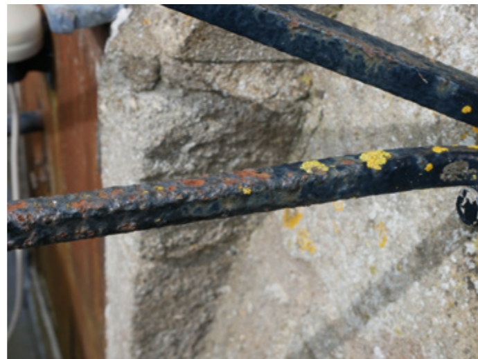
P10 Tower South elevation clock stays
