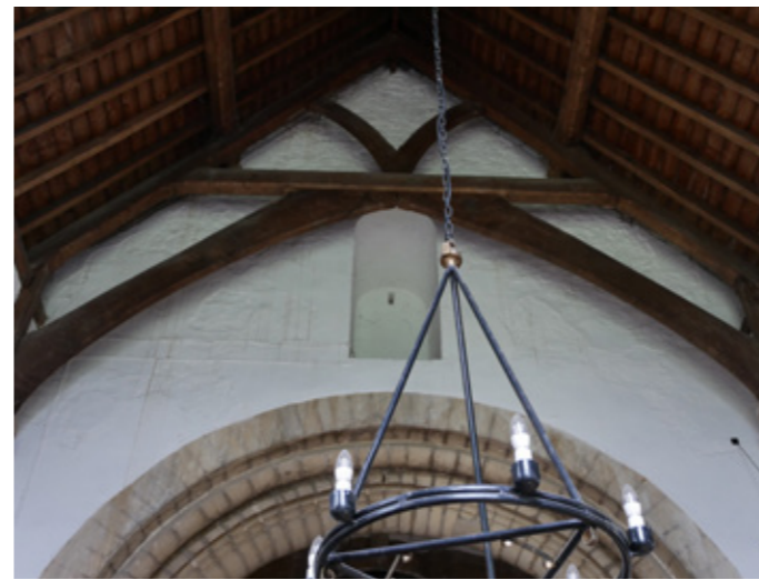
P31 South Transept North wall
