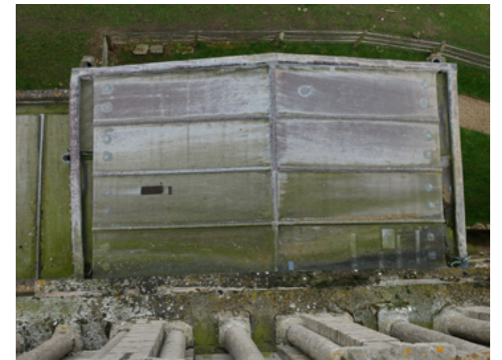
P08 North Transept roof
