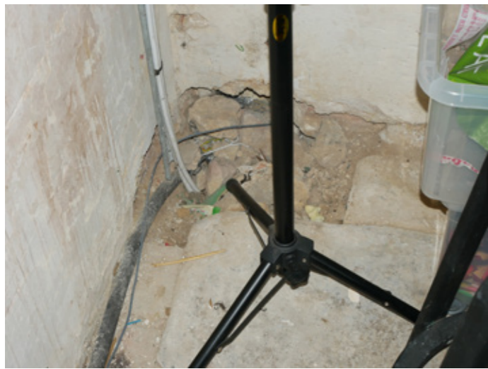
P29 North Transept floor
