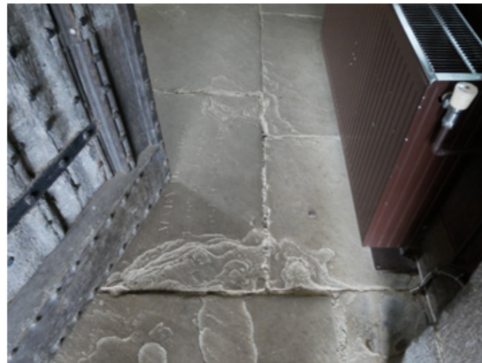
P34 South Aisle floor inside door D1
