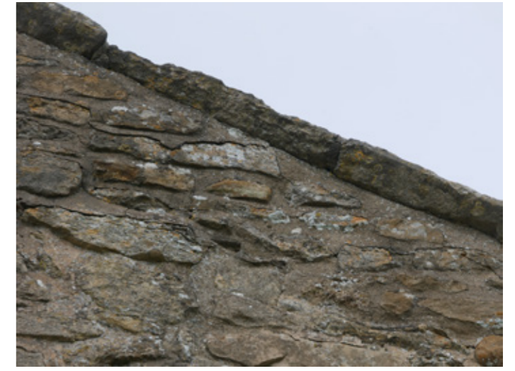
P16 Vestry South elevation coping
