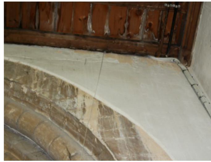
P27 North Transept South West corner
