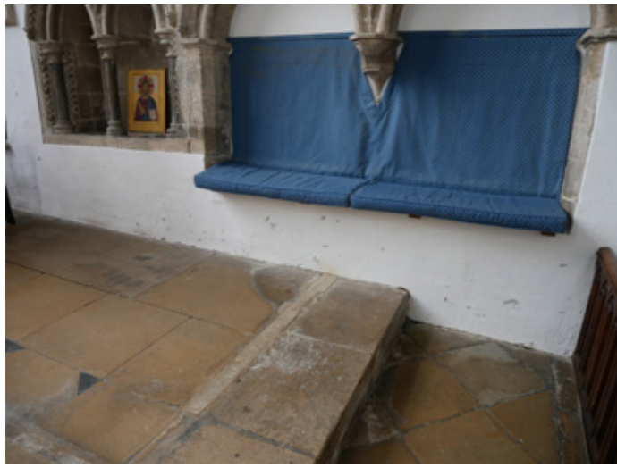
P25 Chancel South wall below sedilia
