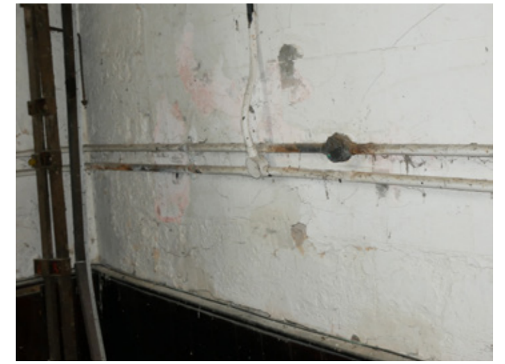
P28 North Transept East wall
