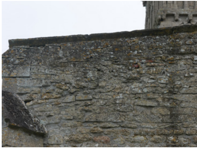
P13 North Aisle West elevation high level
