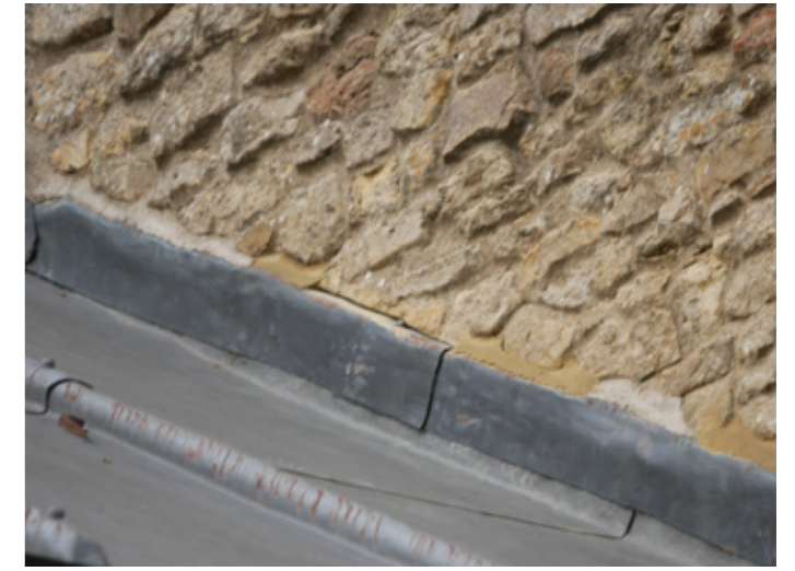
P04 Vestry roof North abutment
