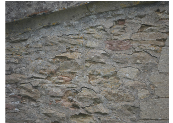
P12 Nave West gable high level mortars
