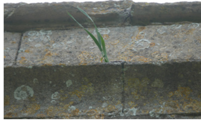
P15 Chancel North elevation parapet
