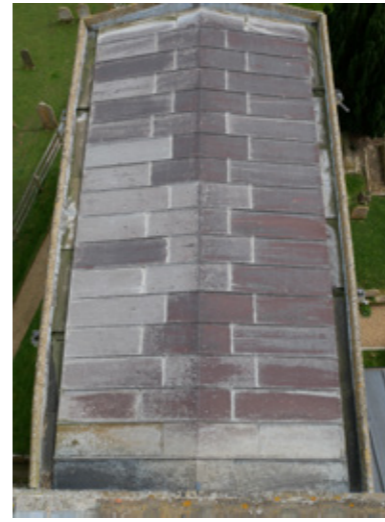
P03 Chancel roof
